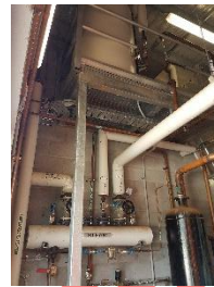
Steam Manifold / Blow-down Vessel / Feed Water tank
