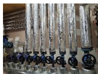
Low Pressure 400kPa Steam Manifold
