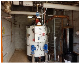
50HP NG-fired vertical Steam Boiler 1000kPa / Steam Meter assembly
