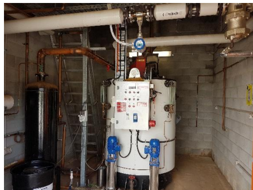
50HP STEAM BOILER, BLOWDOWN VESSEL, STEAM METER,
